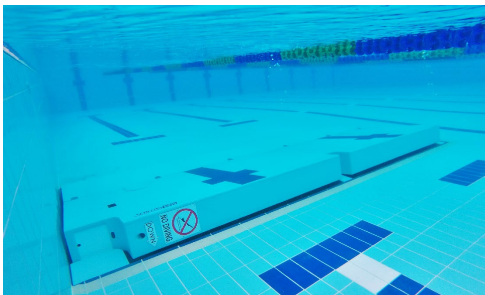
Figure 5. SwimWall segment lowered to pool bottom.
