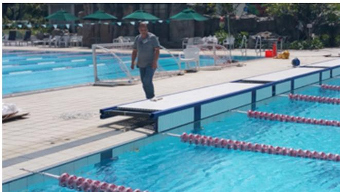
Figure C: The EndWall sections are assembled and connected together on the pool deck. The Support Legs and Anchor Legs are placed under the EndWall for support, but are not fixed into place yet.
