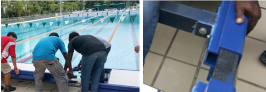
Figure A: Connecting the EndWall sections together with the Connector Sleeves (image on right).
